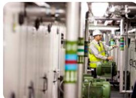
Christie Hospital – AHU Replacements £0.3m (M&E)
