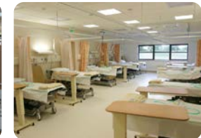
Leighton Ward 6 Refurbishment £1.0m (M&E)
