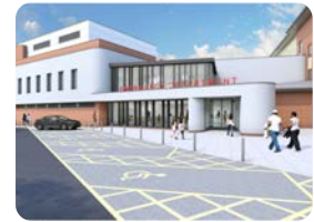
Wythenshawe Emergency Department Upgrade £4.3m (M&E)
