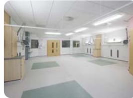
QE/Good Hope/Heartlands - Ward Upgrades £4.7m (M&E)
