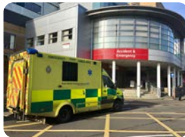
Yeovil Hospital Emergency Department Reconfiguration £1.0m (M&E)
