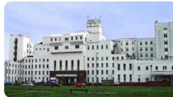
Epsom & St Helier University Hospital Rapid Works £0.2m (M&E)
