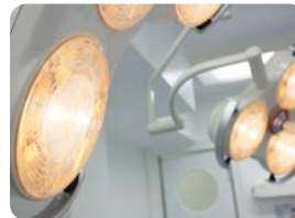
Prince Charles Hospital Theatres £2.0m (M&E)
