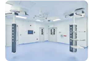
Queen Elizabeth Hospital - Theatre Refurbishment £3.5m (M&E)
