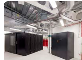
Yeovil Hospital – Lighting, Fire Alarm, IPS/UPS £2.0m (M&E)
