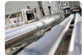
County Hospital Stafford Domestic Water & AHU £0.8m (M&E)
