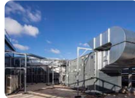
Prestwich Hospital - M&E Infrastructure Upgrades £0.3m (M&E)
