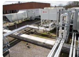
County Hospital Stafford AHU Replacements £0.6m (M&E)
