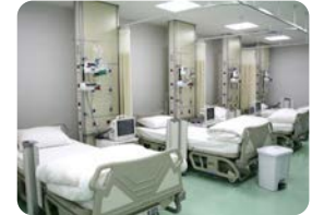
Royal Preston Hospital - Ribblesdale Ward £1.0m (M&E)
