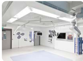
Leighton Hospital Theatres £8.5m (M&E)
